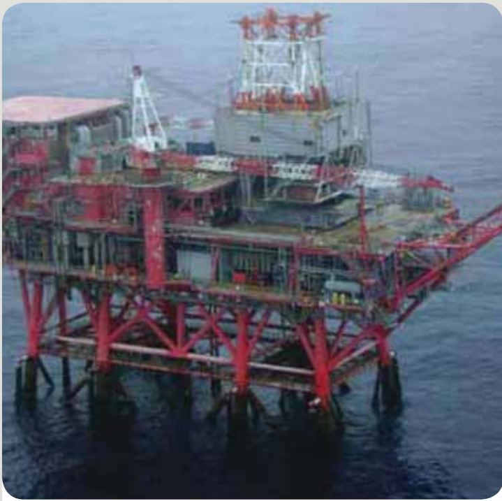
One of the IWAKI platforms prior to decommissioning.
